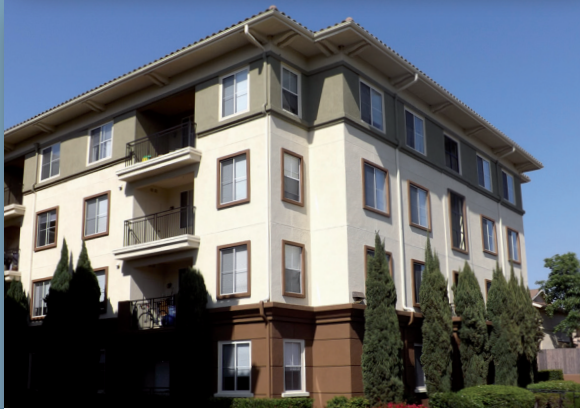
HOA & Commercial Stucco Repairs & Application
