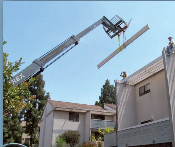
Wood Repairs & Replacement
