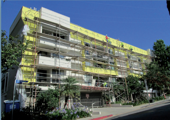
HOA & Commercial Defect Repairs
