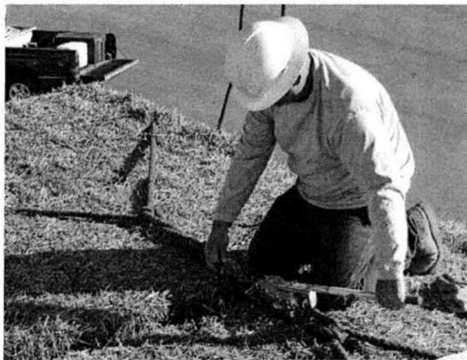
Figure 2. Locking Tightener (Binder)
